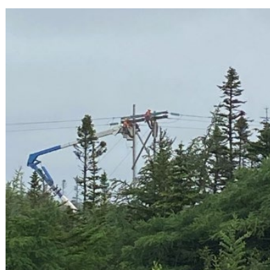
Crews making repairs to transmission line 55L that was damaged by lightning.
