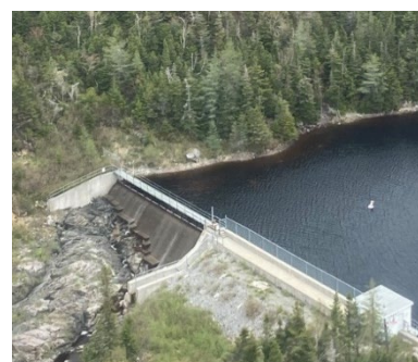
Lookout Brook Hydroelectric Generating Plant forebay dam and spillway.
