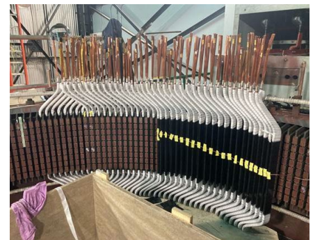
Stator coils at Sandy Brook Hydroelectric Generating Plant.
