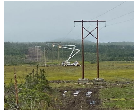
H-frame structures under construction on transmission line 94L.
