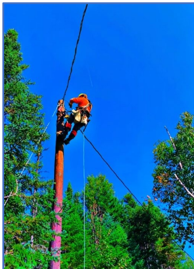
Crews connecting a new residential service in a wooded area near Grand Falls-Windsor.
