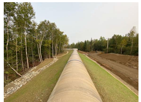
New penstock at Sandy Brook Hydroelectric Generating Plant.
