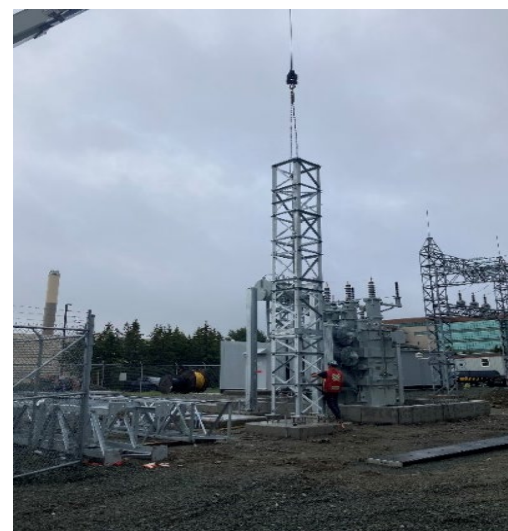
New transformer and structures at Long Pond Substation.
